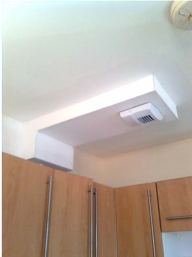
Duct and moisture / odour sensitive vent
