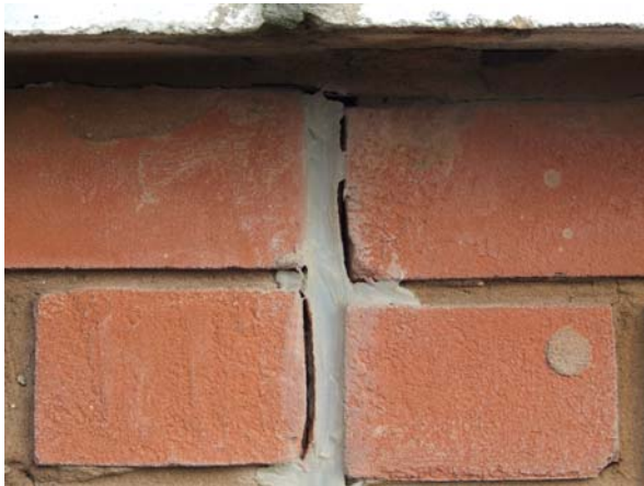
Photograph 10 - Expansion joint in brickwork with mastic infill material
