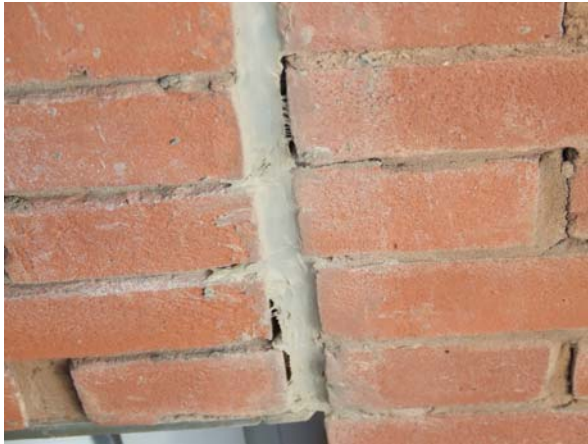
Photograph 9 - Expansion joint in brickwork with mastic infill material
