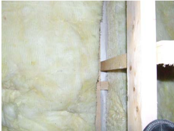
Photograph 31 – Gap and spacing between insulation layers within the main attic
