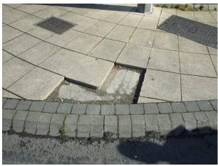
• The kerb to the front gardens and entrances are not suitable for wheelchair users because the level difference is in excess of 50mm.
