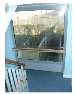
• The handrail in front of the windows at landing is not acting as a barrier or guarding and in one location the guarding is loose.
