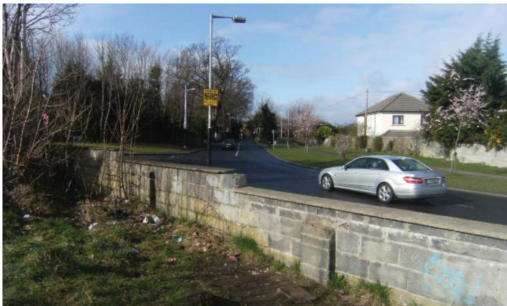
Wall blocking access to Knocklyon Rd
