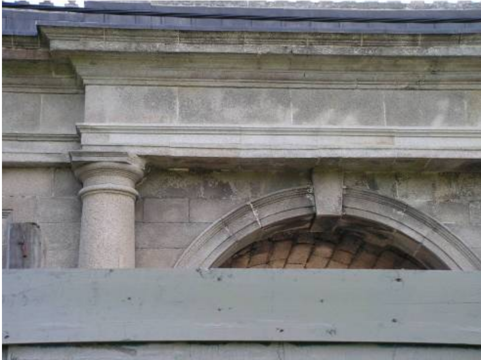
The north-eastern entablature: the completed repair (photographed September 2010)
