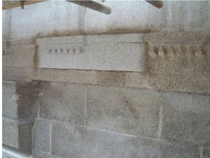
The lower frieze of the south-western façade: the completed new granite lintel.
