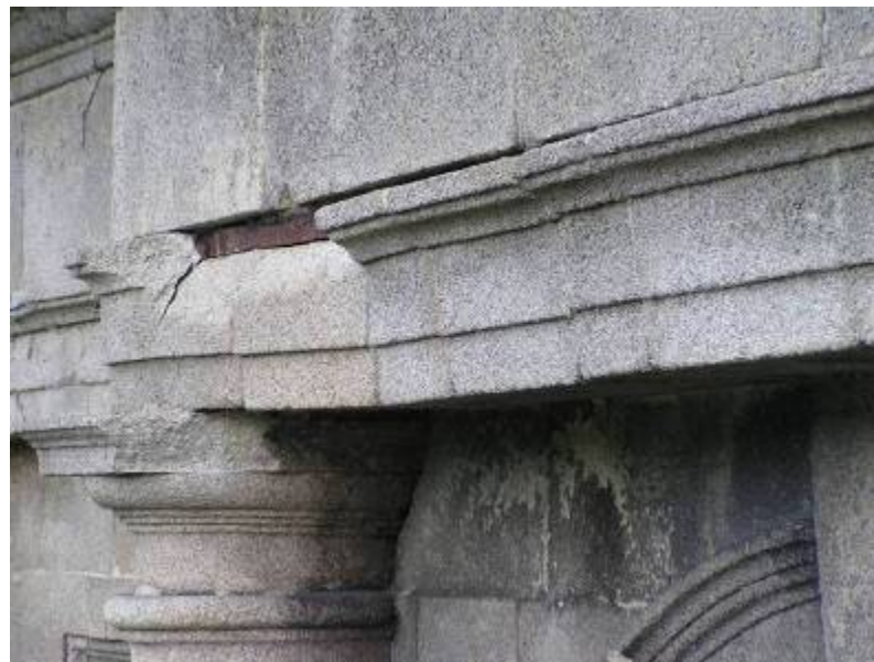
The architrave of the north-eastern entablature before the works began
