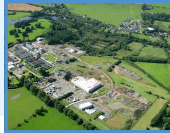
Ballymore Eustace Water Treatment Plant
