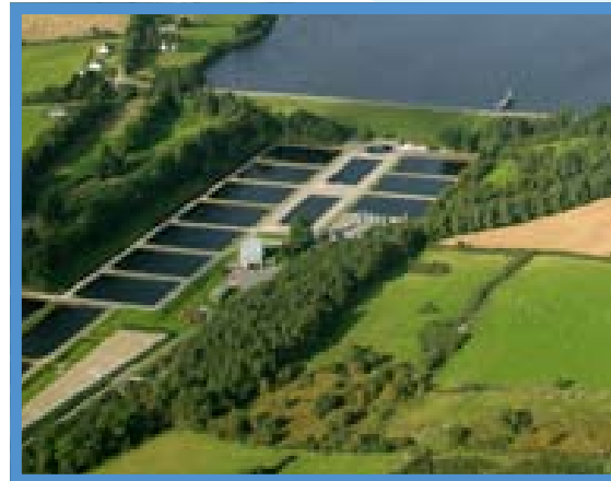
Vartry Reservoir and Water Treatment Plant
