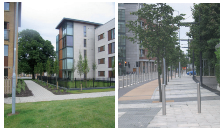
Fig. 24 Supervised pedestrian route in Adamstown.
