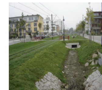
Fig. 42 SUDS adjoining grass tram track, Vauban.
