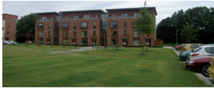
Fig. 28 Semi private amenity space in Adamstown. Parking is only on two sides.
