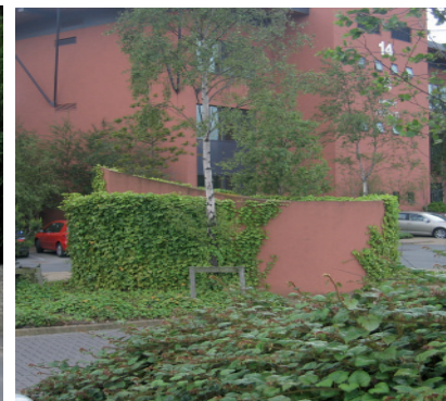
Fig. 8 Offices in Citywest
